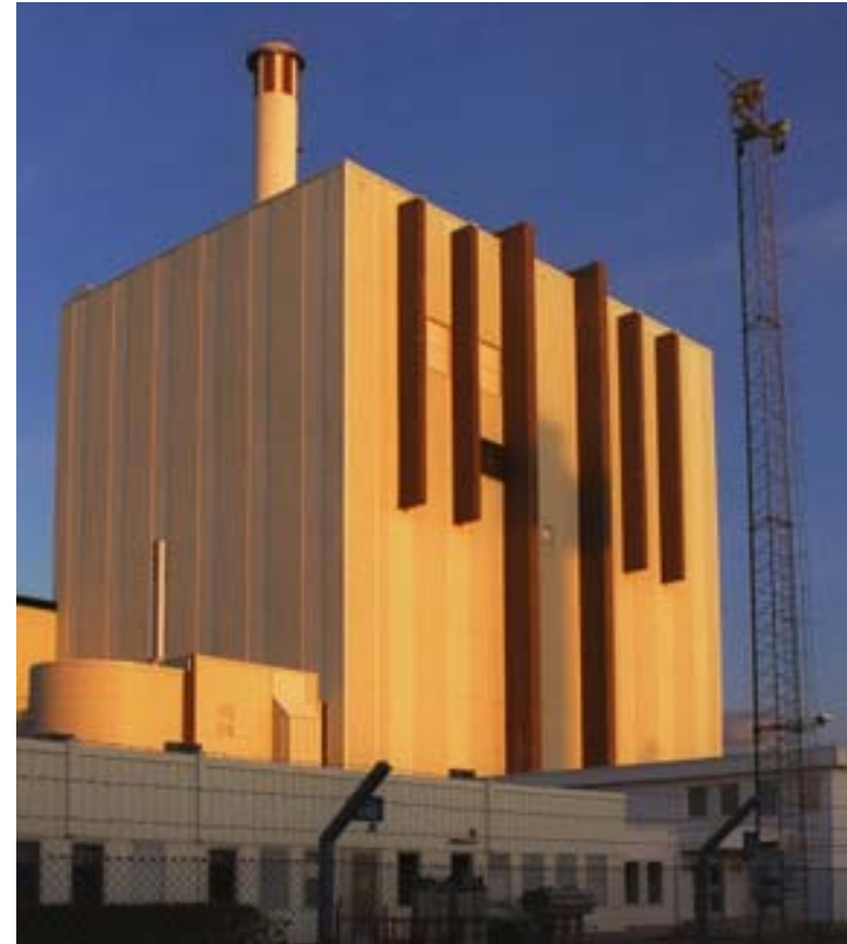
Forsmark Nuclear Power Plant, Sweden
