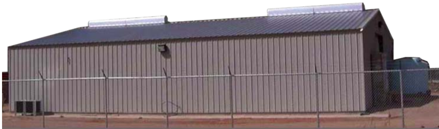
Vanadium Redox Battery, Source: Cellstrom GmbH
